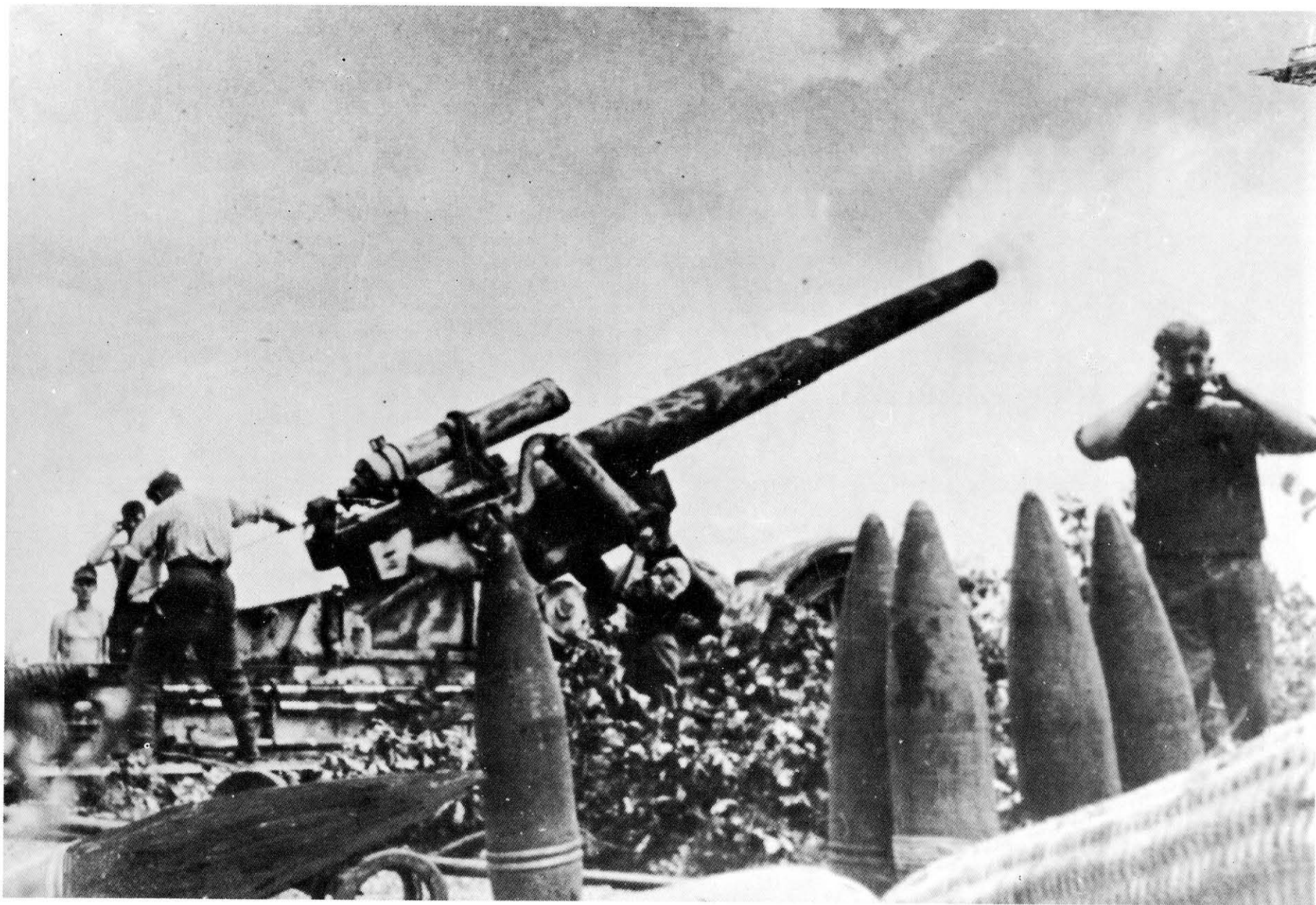
21cm Msr 18 firing in the lower elevation group in Russia, September 1943. HE and concrete-piercing shells can be seen in the foreground, ready for the next salvos. The 100kg shells smash into their target with an initial velocity of between 225-565 meters per second.
